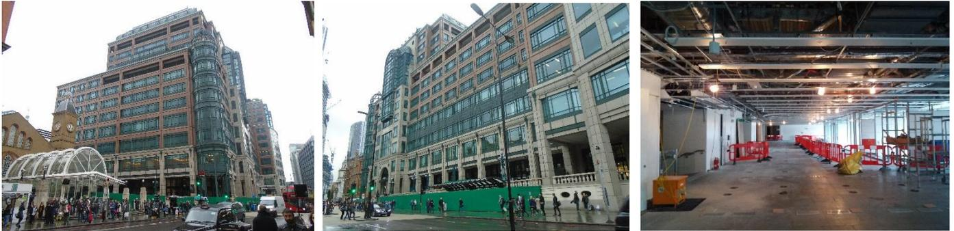
Cantillon's scope includes the management and isolation of all M&E, asbestos removal, soft strip, facade removal and structural alterations. Work began on site in September 2017 and are due to complete in April 2018. During the early stages of the project the scope was increased to include the removal of all redundant plant and plant rooms at ground floor level. This phase 2 work is to be completed within the same programme as phase 1.
