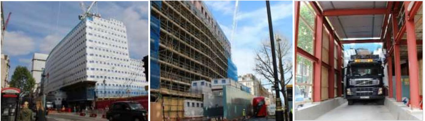
Allied with delivering against these constraints, Oxford Street situated to the North, represented the only opportunity to service the site and involved the removal of nearly 15,000t of demolition materials, loaded using alternative methods to avoid requirement for HGV Lorries crossing the pedestrian footpath on London's busiest street.
