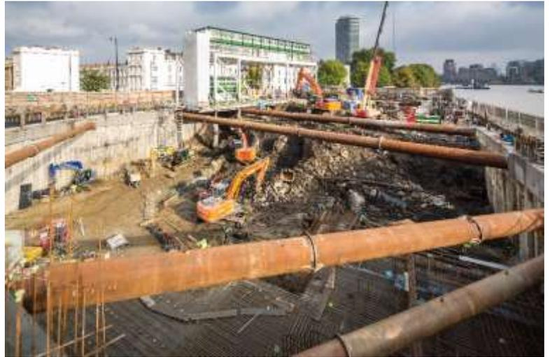
The project involved the demolition of a 13 story office block and a 2 level basement alongside the River Thames in Pimlico. On completion of the demolition, Cantillon worked in conjunction with and attended the piling contractor in advance of undertaking the bulk excavation and propping scheme.
