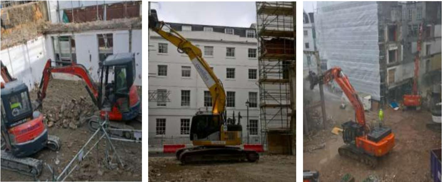
This has enabled Cantillon to get a better understanding of when each neighbouring property might be affected by the nature of the scope of works, in order to take the appropriate robust measures to try and mitigate any impact. The demolition techniques included traditional floor by floor methods, as well as high reach methodologies. Pile testing was undertaken at this stage.
