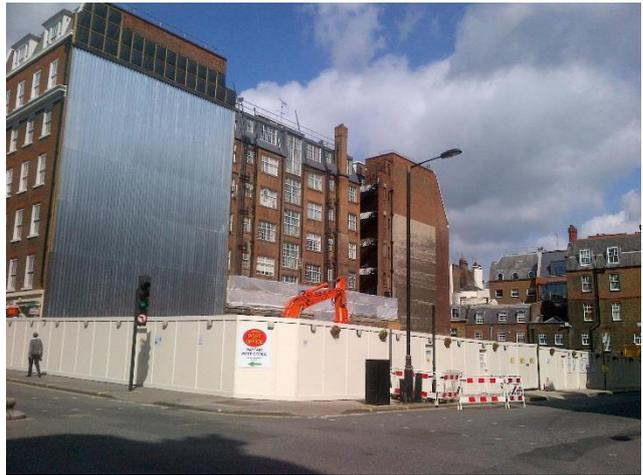
After carrying out a full soft strip of the building back to the shell concurrent with the removal of notifiable and non-notifiable asbestos to every level, Cantillon undertook the structural demolition and clearance of the existing building down to the basement slab.
