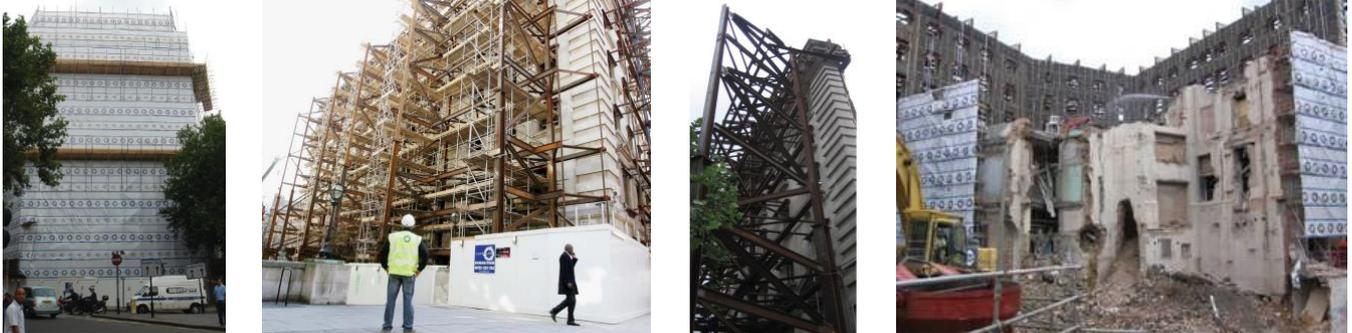
Limited information at tender stage had led to a decision being made to carry out exploratory work to determine the existing foundation type to the façade foundation. These varied work to determine the existing foundation type to the façade foundations. These varied greatly and we designed a continuous ring beam and foundation solution to overcome the problem instead of the mini piled solution suggested by the engineers.
