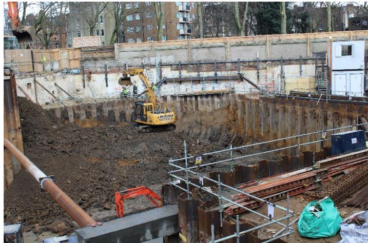
Installation of structural blinding above new formation level was used as a piling mat for ground source heat pump piling and the installation of bearing piles for the construction of the tower crane bases.
