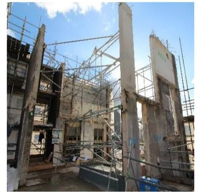
Cantillon scope included asbestos removal, soft strip, facade removal, structural alterations, piling and underpinning. Work began on site in July 2015 direct with the client, a pre-agreed novation to main contractor Wates, occurred in February 2016. Works are due to fully complete in June 2016.
