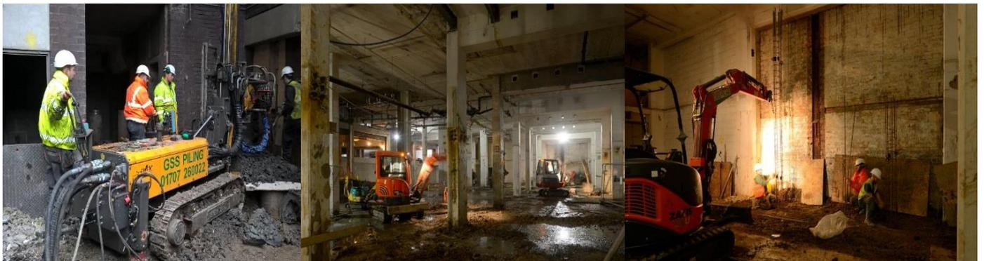
Slots through the RC slabs were diamond cut and then broken out. Some pile locations also had nominal horizontal clearance to adjacent structure. Out of the 54 piles over a third were constructed using a Super Kitten rig, the remainder with a Klemm 702. Concrete to the piles was fed from a pump via a static line. These, and the drainage enabling works, were completed on time for the main contractor.
